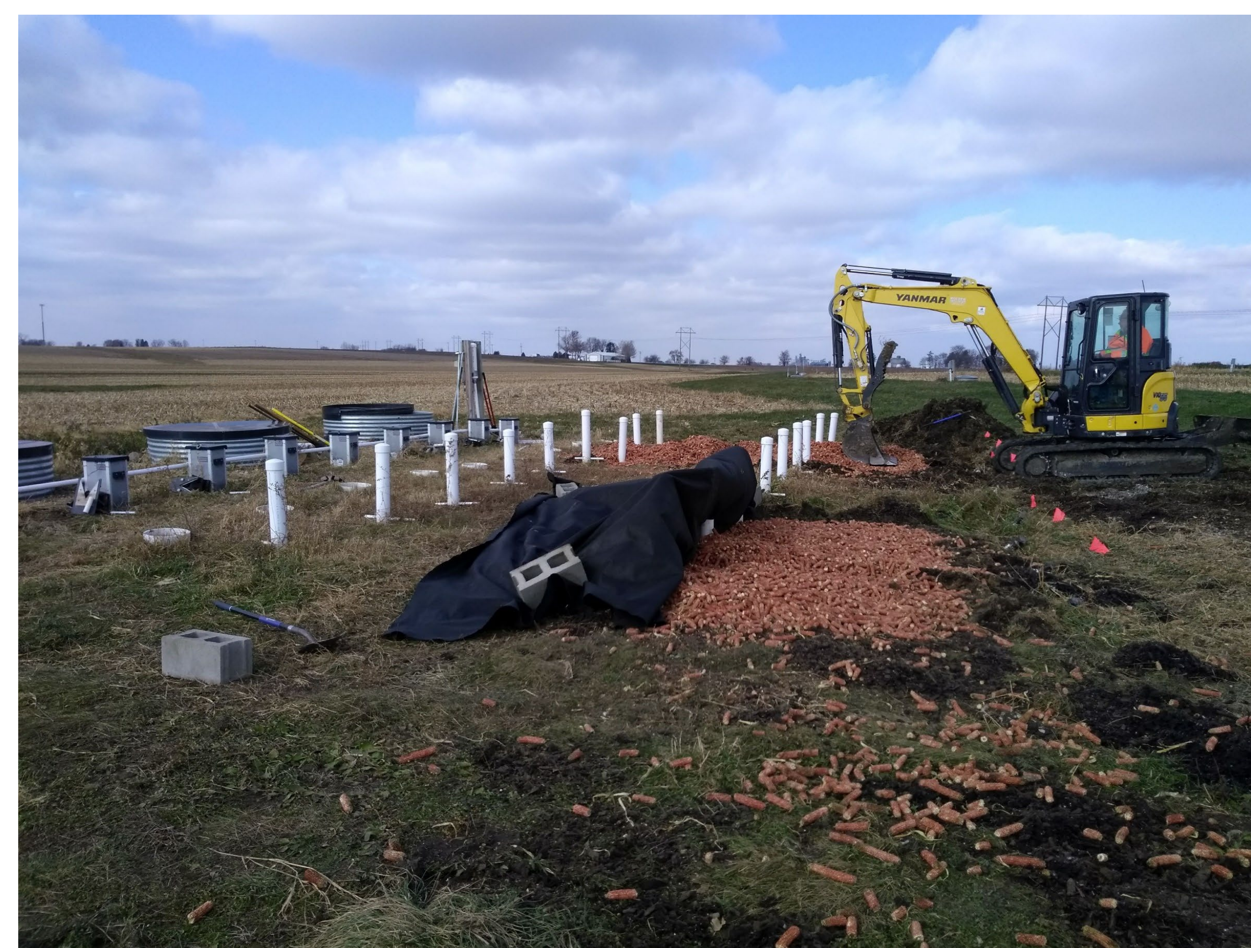
Construction of nine pilot scale woodchip bioreactors at Iowa State University
